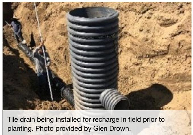
Tile drain being installed for recharge in field prior to planting. Photo provided by Glen Drown.
